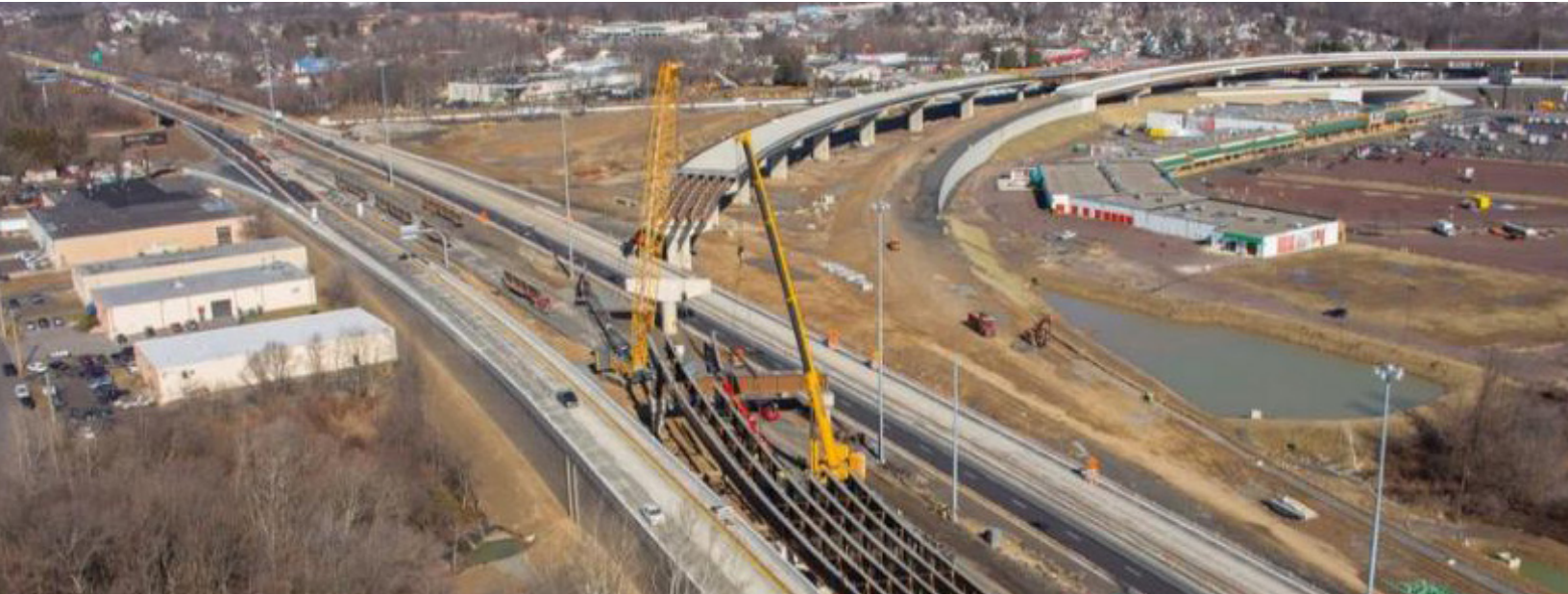
Construction of the PA Turnpike/I-95 Interchange, Bucks County
